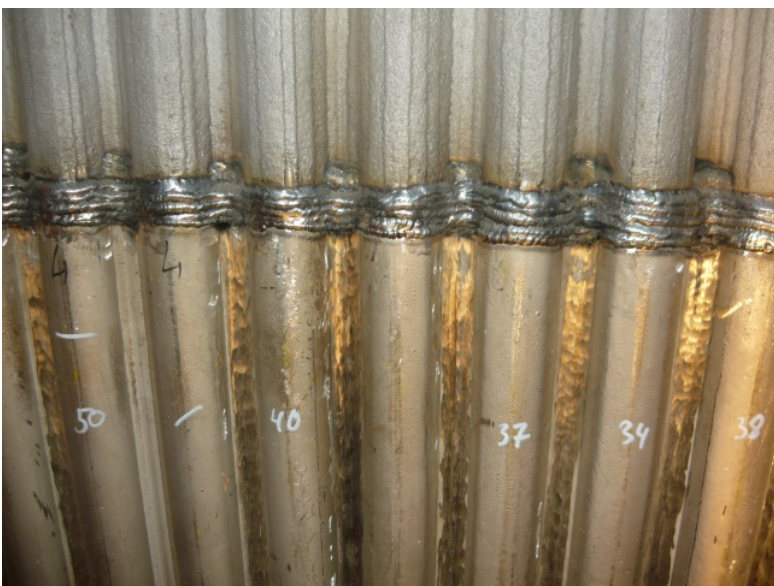
Abb. 2-3: Paneelstoß an "Alt-Inconel"
