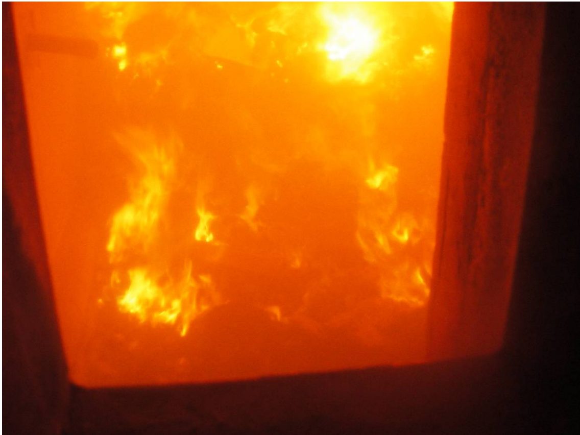
Figure 3.12: Instability with “long fire” and high bed height photographed from the deslagger side of the combustion chamber
